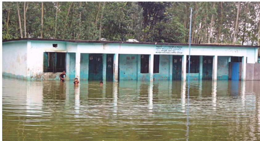
Figure 5.6: Flood affected educational institute Source: Google Image
