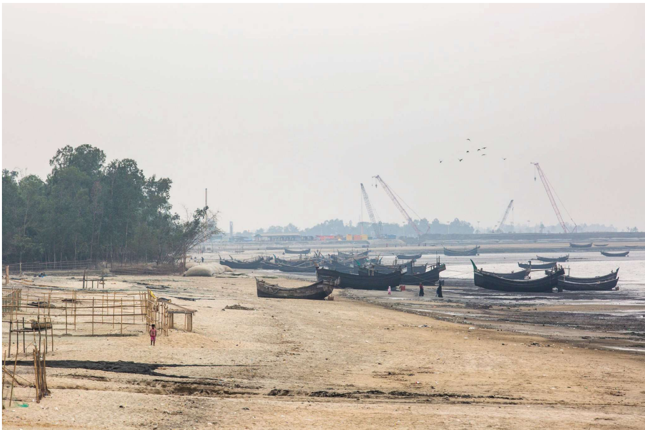
This fishing community village is a stone's throw away from the under construction Matarbari 1 coal power project. Photo Credit: Market Forces
