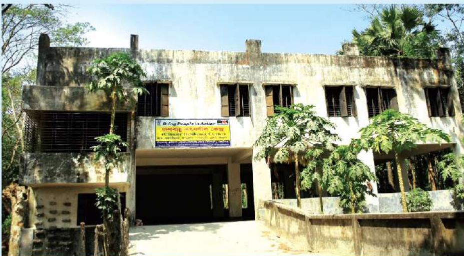
Traditional Cyclone Shelter is being used as Community Resilience Center
