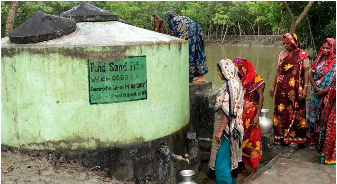
Women are collecting potable Water from their own managed Pond Sand Filtration (PSF) Plant
